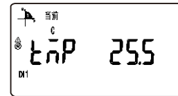
Voltage on A phase is Temperature on T3 is 25.5 cent degree123.4V
